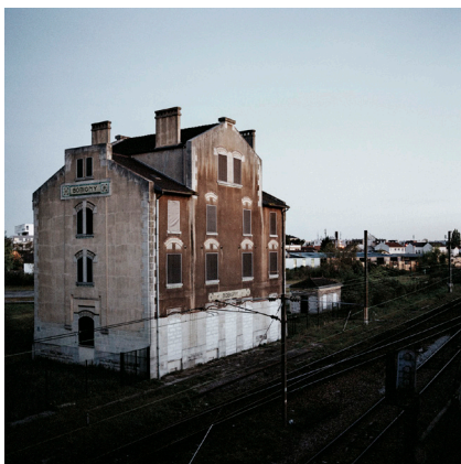
Former Bobigny deportation station Paris, France, 2016
